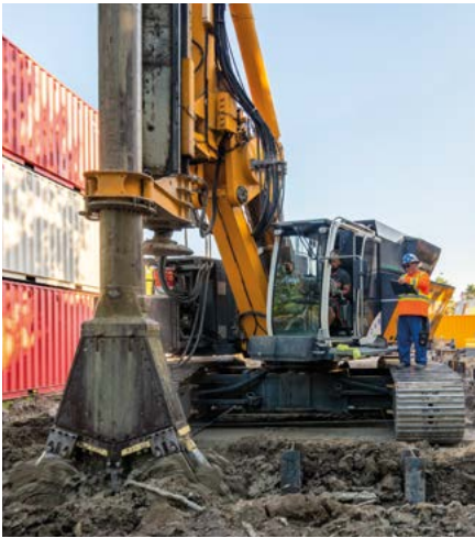
BCM 5, Verbauwand, Niederlande BCM 5, Retaining wall, Netherlands
