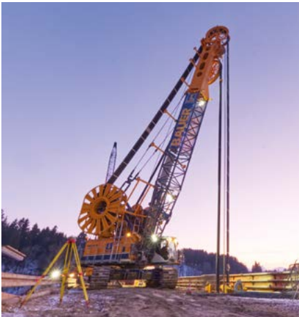
MC 96 / BC 48, Dichtwand, Deutschland MC 96 / BC 48, Cut-off wall, Germany
