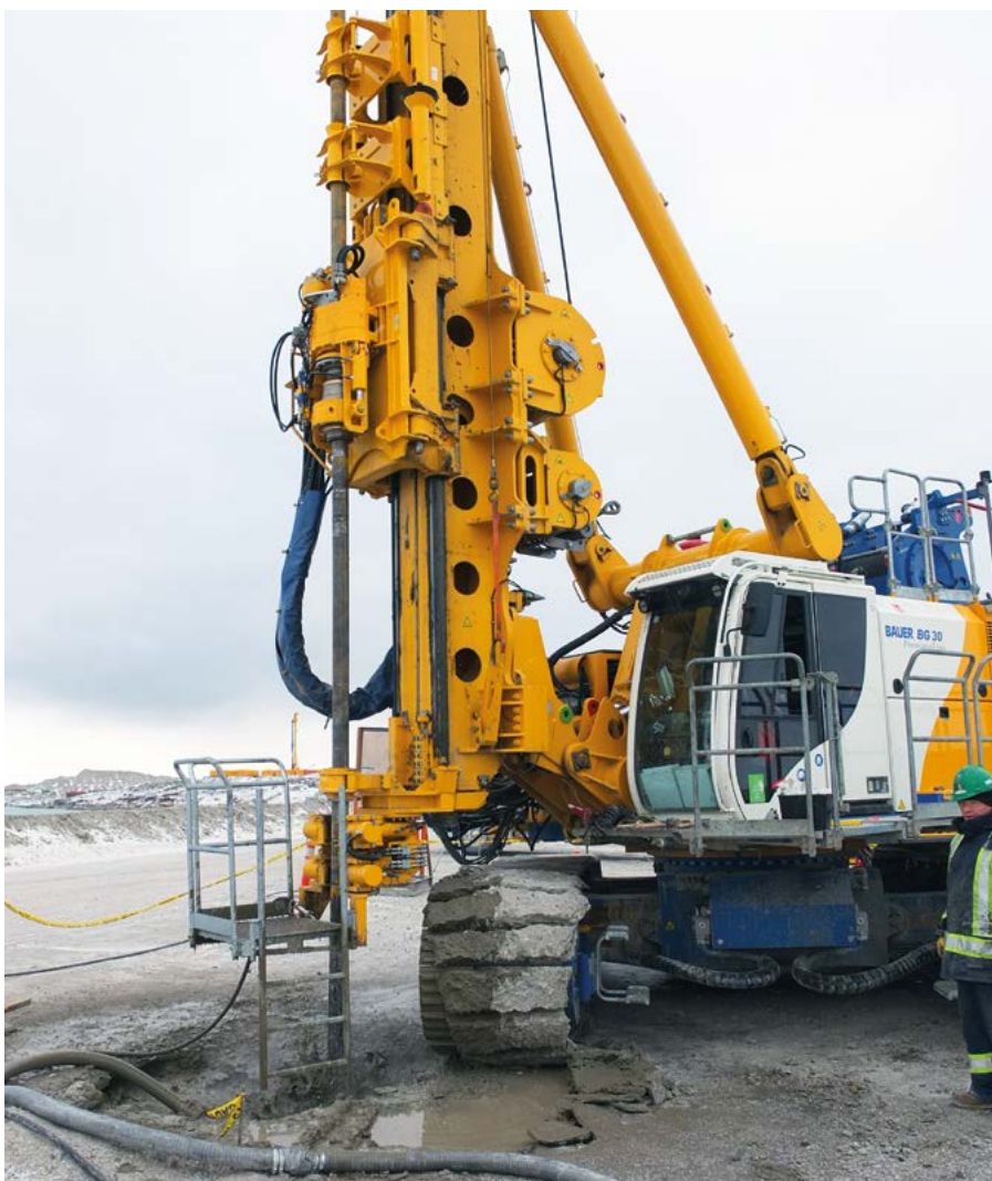
BG 30, Dichtwand, Kanada BG 30, Cut-off wall, Canada
