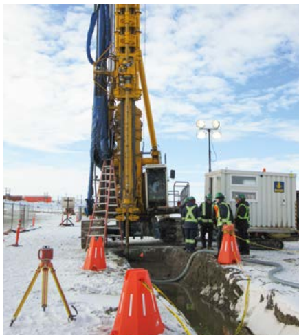
BG 30, Dichtwand, Kanada BG 30, Cut-off wall, Canada
