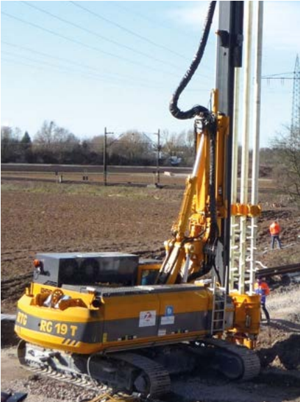
RG 19 T, Dichtwand, Deutschland RG 19 T, Cut-off wall, Germany
