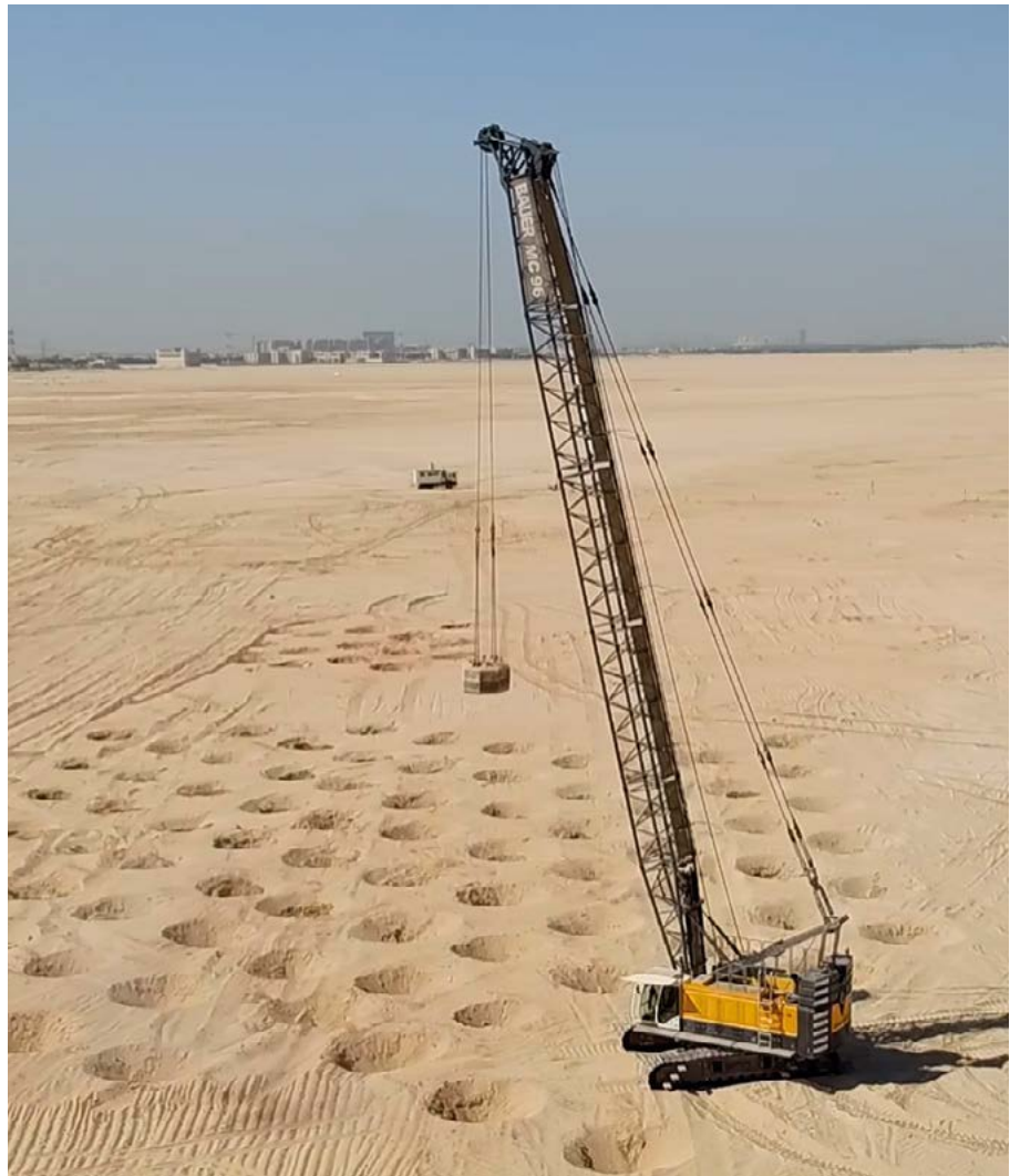
MC 96, Bodenverbesserung, Abu Dhabi MC 96, Soil improvement, Abu Dhabi
