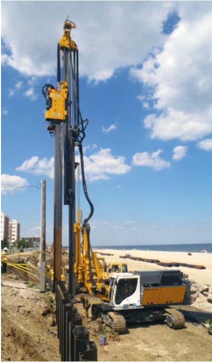
RG 19 T, Rütteln, USA RG 19 T, Sheet pile driving, USA
