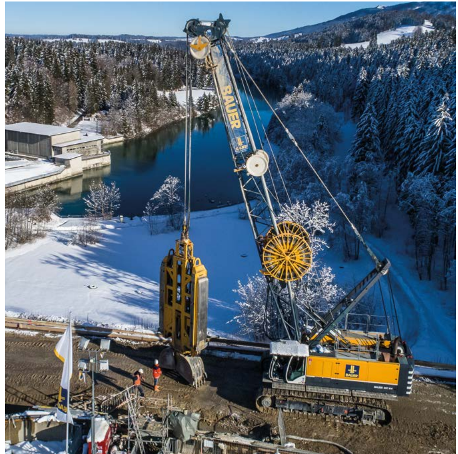
MC 64 DHG-V, Dichtwand, Deutschland MC 64 DHG-V, Cut-off wall, Germany
