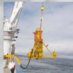
2011/2012 Monopile foundation in rock for tidal turbine with BSD 3000 (Orkneys, UK)
